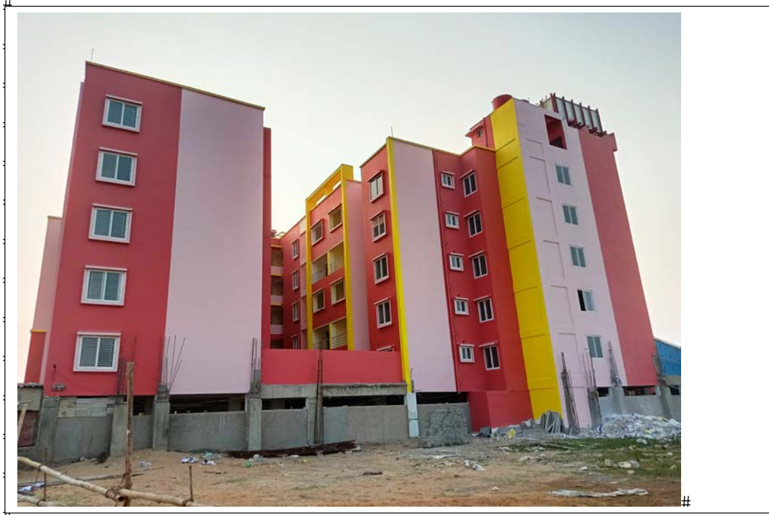
Block A (Part ) : Progress 90%
