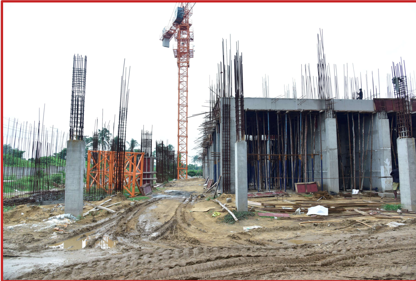
Basement Slab Casting Complete
